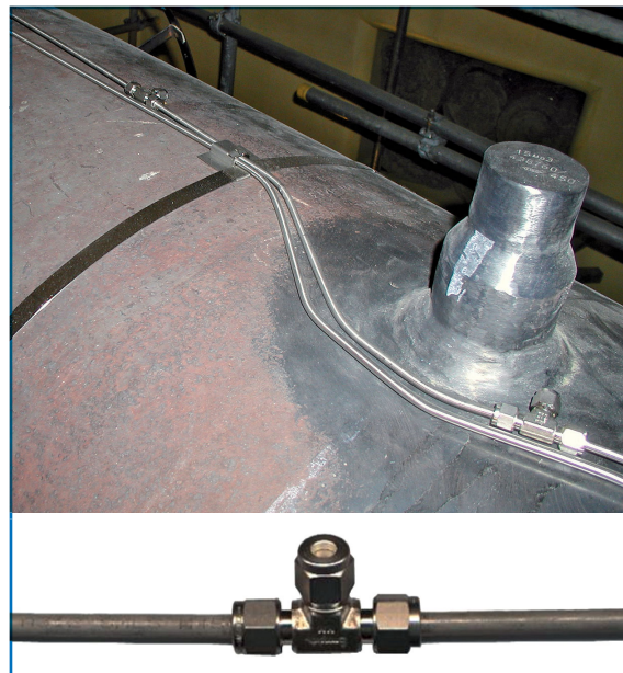
Leakage monitoring on the main steam pipe using humidity-sensing elements
