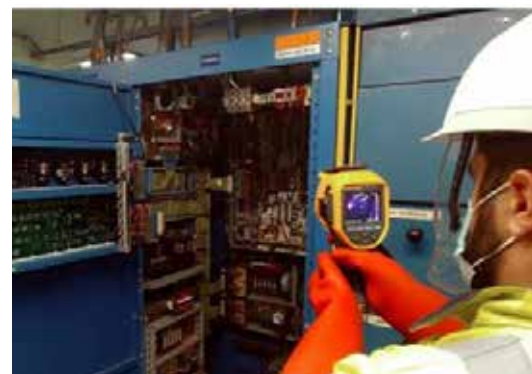
Thermography in the process of being carried out on an inverter
