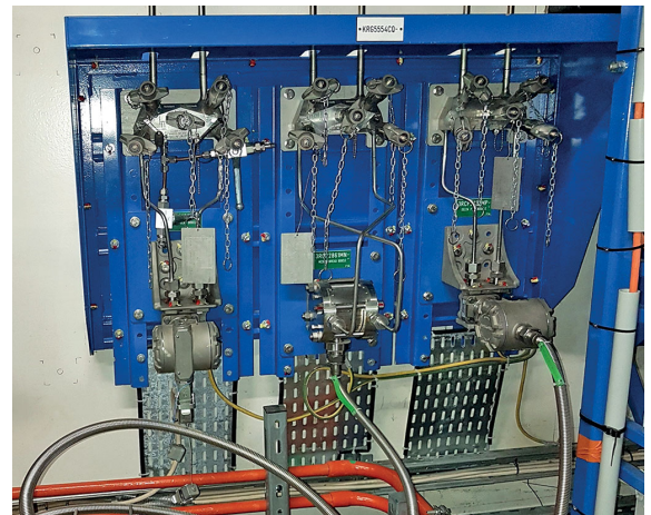
Pressure measurement and level installed in primary circuit
