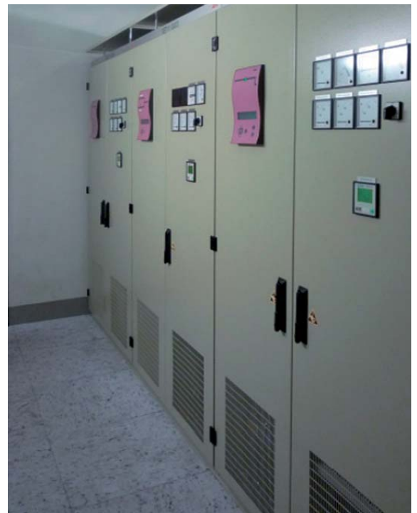
Nuclear Power Plant Gösgen (Switzerland): Two inverters (170 kVA each) and a STS (bypass)
