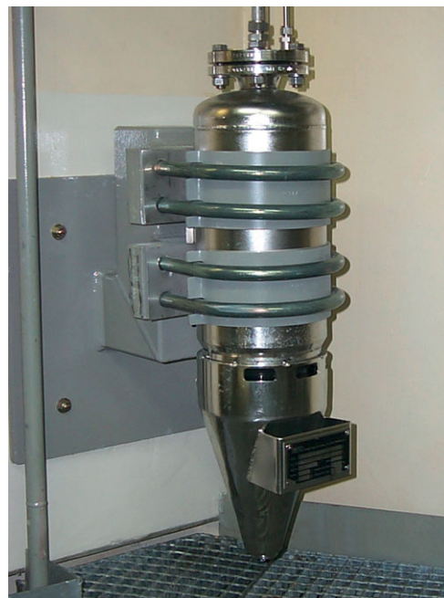
Pool sampler installed inside the containment
