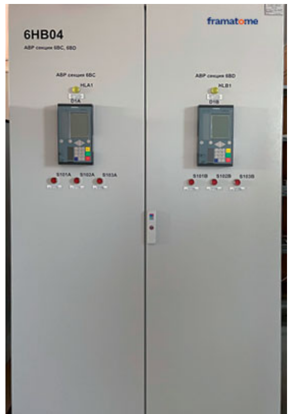
Cabinet for high speed busbar transfer system
