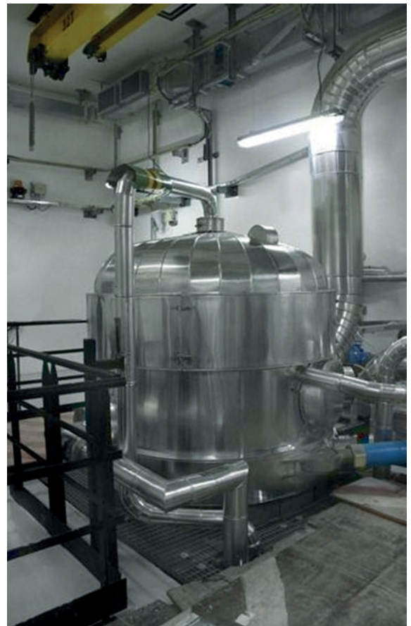
Installed evaporator unit
