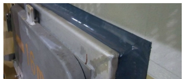
Sealing of wall penetration in an epoxy painted reactor cavity
