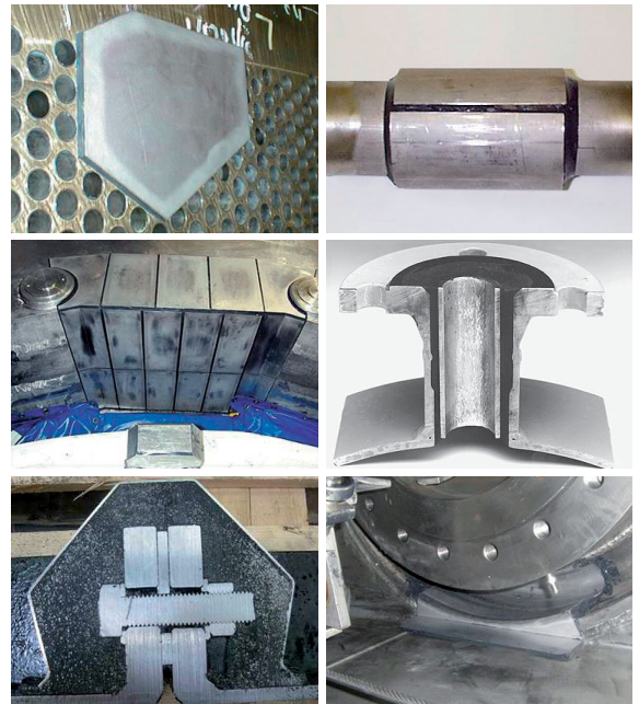
Repair examples: tubesheets, retaining clamps, lining, pipe nozzles, flanges and expansion joints
