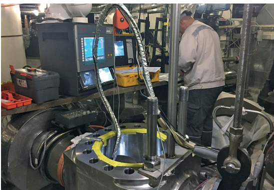
Mechanized welding remote controlled in the valve
