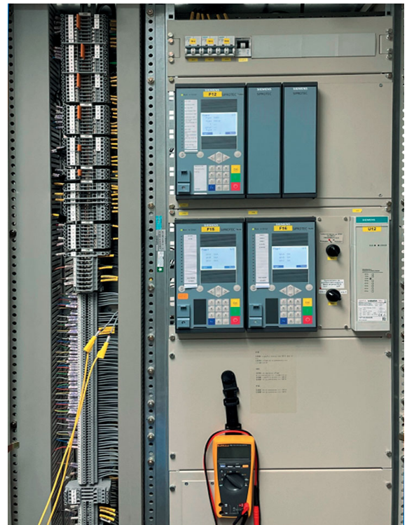
Installation and Testing in the field
