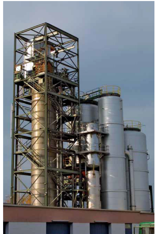
INKA test facility, Karlstein, Germany
