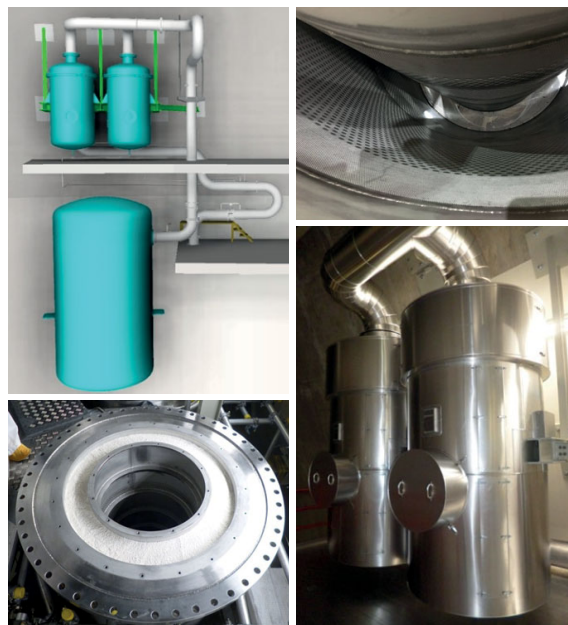
... picture of installed retrofit solution...
