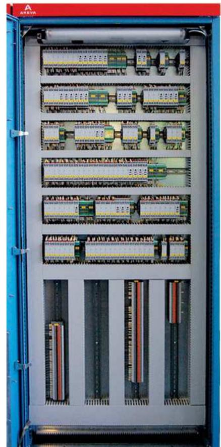
Example of a relay-based analog EDG safety control cubicle
