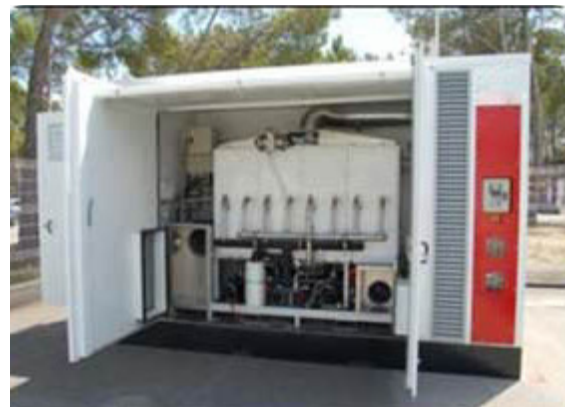
Framatome's 100 kVA MISTRAL Fuel Cell back-up power system
