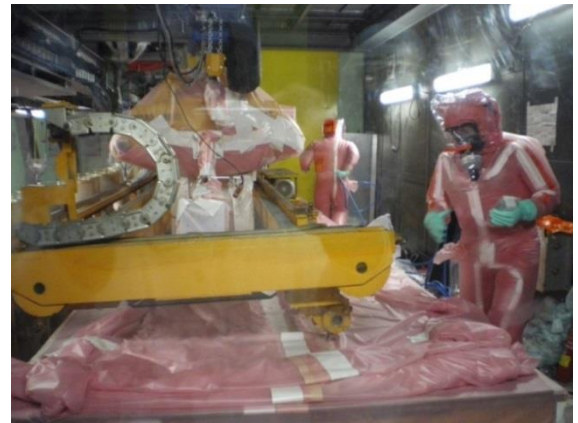
Replacing a lifting unit in a hot cell (Phenix)
