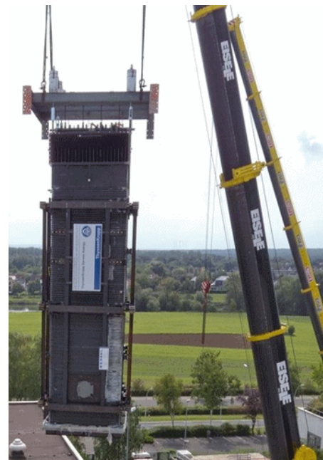
Arrival of the new Benson boiler
