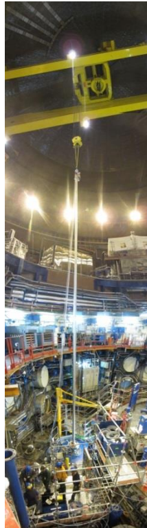
Introducing a drainage tool in the vessel
