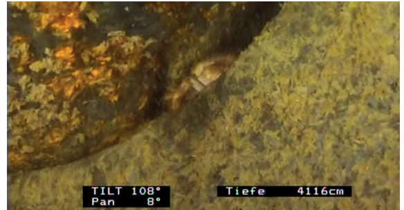
Inspection camera image
