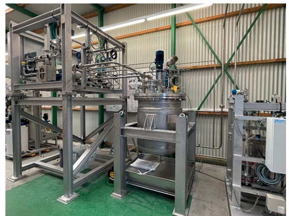
Set-up of the test facility at Framatome site in Karlstein am Main, Germany
