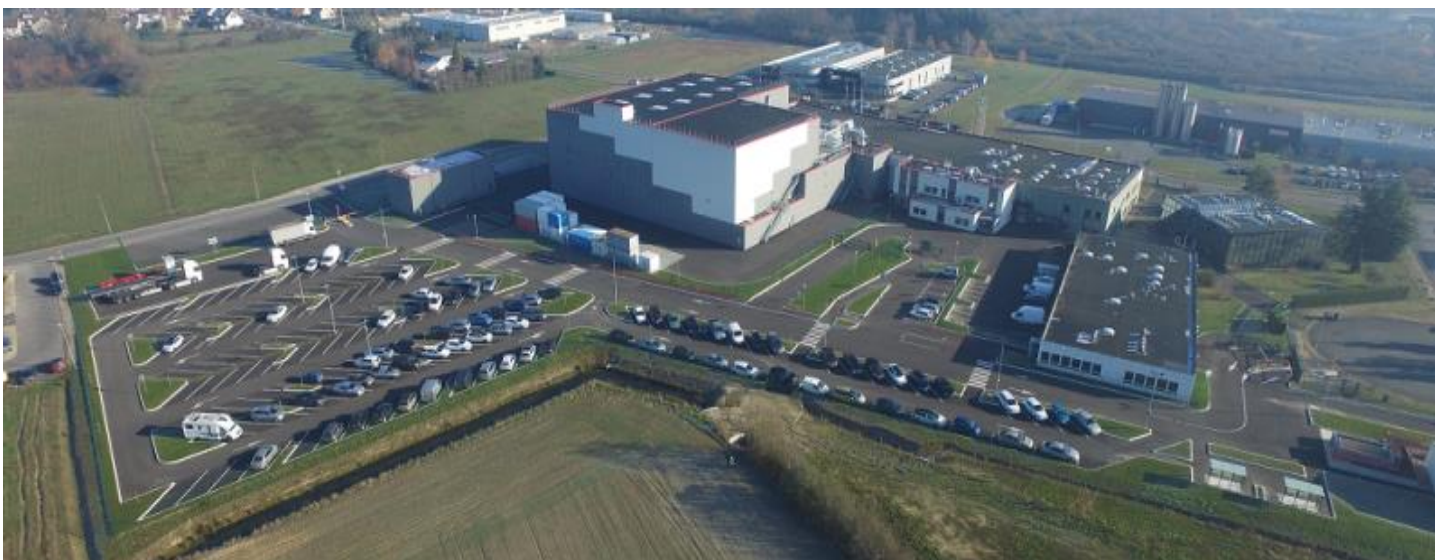
CEDOS hot workshop at Sully sur Loire
