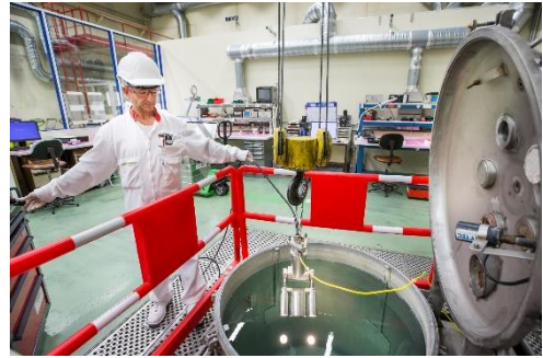
Maintenance workshop in the Framatome controlled area ©
