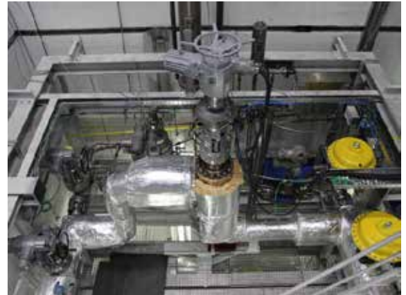
Qualification test of a valve
