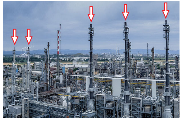
Monitored chemical plant structures
