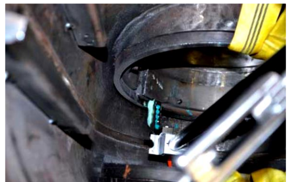
Investigation of a valve inaccessible with conventional methods
