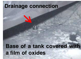
Internal view after complementary drainage of tank MAS0 01BA
