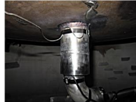
Connection welded to the base of a tank
