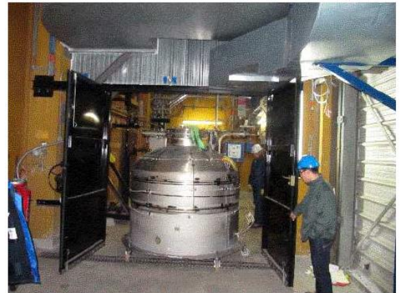
Inserting a tank in the TND draining facility
