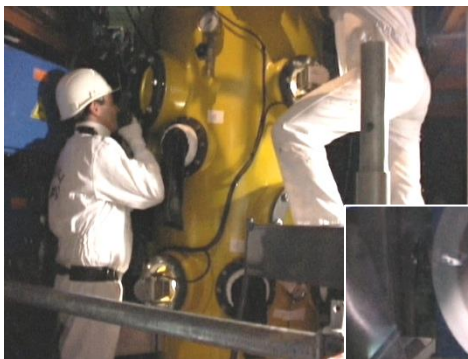
Drilling of the Super-Phenix corium recovery system under 15 m of liquid sodium
